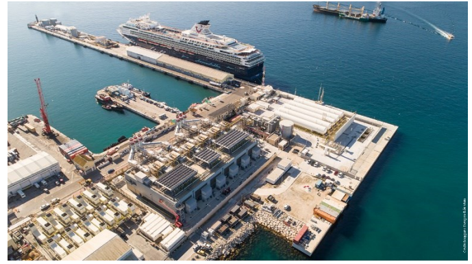
Figure 9-5, Interplay between ICE Power Plant of MAN SE and LNG terminal in the port of Gibraltar
