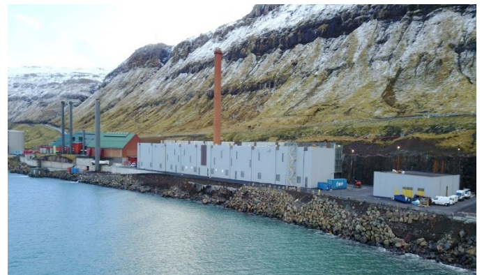
Figure 9-2, ICE Power Plant of MAN SE is a part of the microgrid of the Faroe Island energy system. The isolated energy system in the Faroe Islands is an impressive example of how all available energy resources can be integrated into an intelligent and innovative microgrid.
