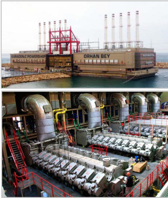
Figure 9-3. ICE power plant. Floating or onshore ICE power plants can be used in the bays near the offshore wind turbines. When there is no wind, these can produce electricity from the stored hydrogen and thus compensate for the resulting lack of electricity in the network and greatly reduce or avoid fluctuations in electricity production.
